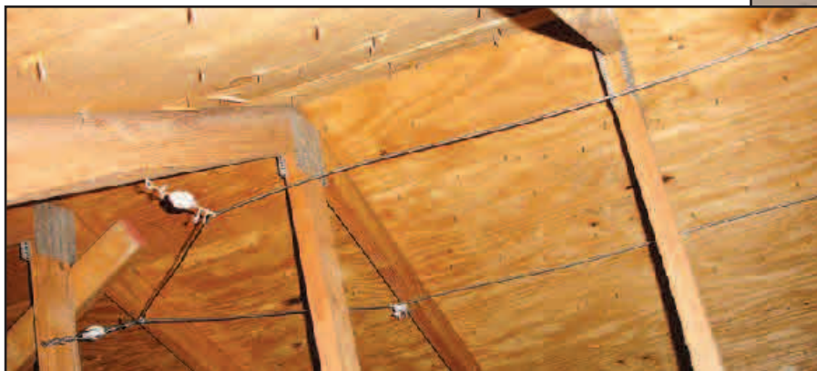
Figure 2 — The inverted L element is supported by egg insulators suspended from the rafters in the attic.
