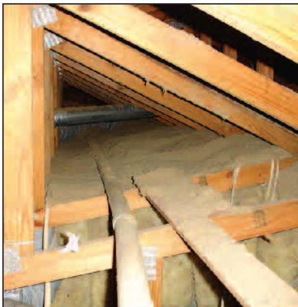
Figure 4 — The ac conduit parallels the antenna elements.
